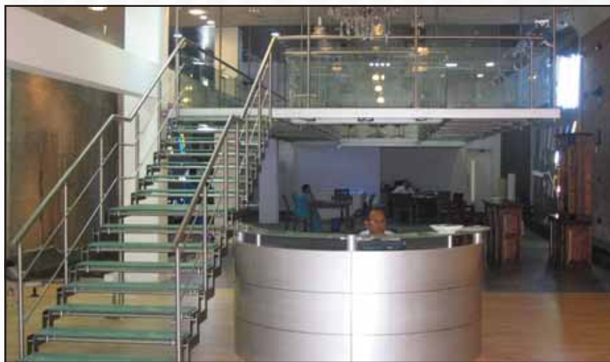
Stainless steel hanging floor in a showroom
