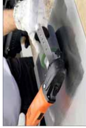
Surface sanding with elastic sanding sleeve Grit 60 with 900 rpm
