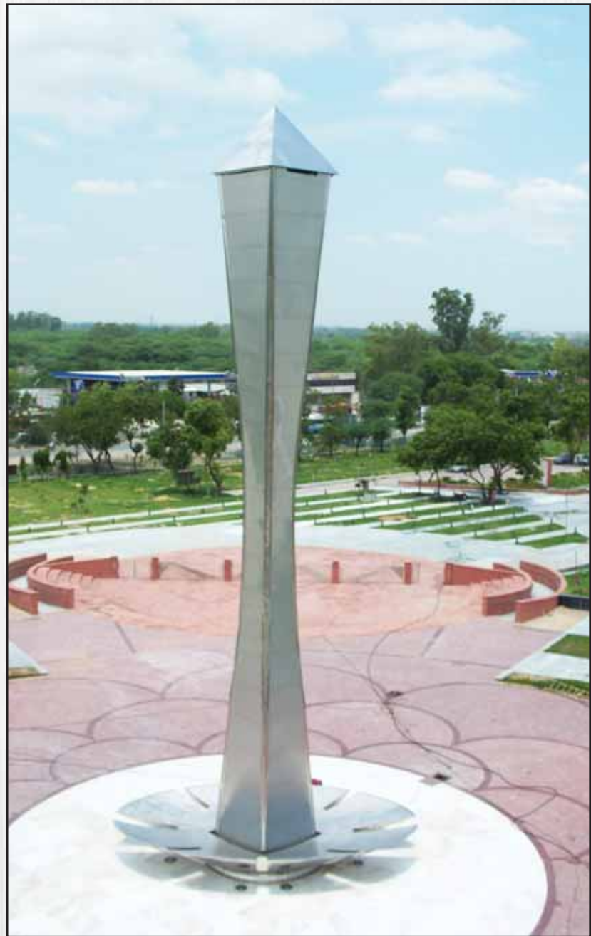
Central Pylon clad in stainless steel is 24 meters tall. The Lotus is elliptical with a mean diameter of about 8 meters.
