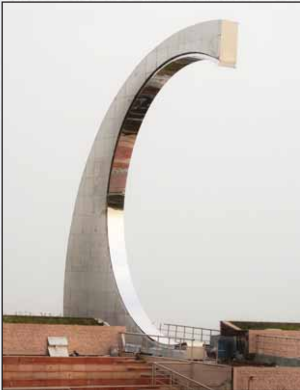
One of the three Semi Arches, 15 meters tall, with stainless steel cladding
