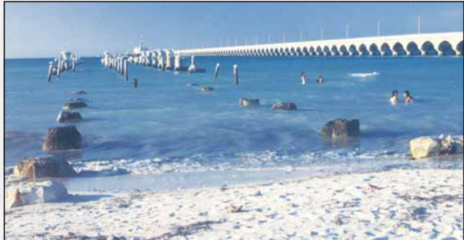
Tale of two bridges at Progresso in Mexico, A study in contrast
