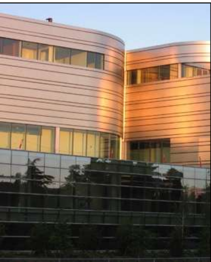
US Federal Courthouse Eugene, Oregon, USA US Gold LEED, 100 year life
