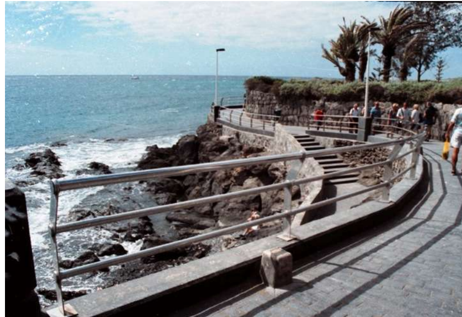
2205 Railings, Canary Island 30 years
