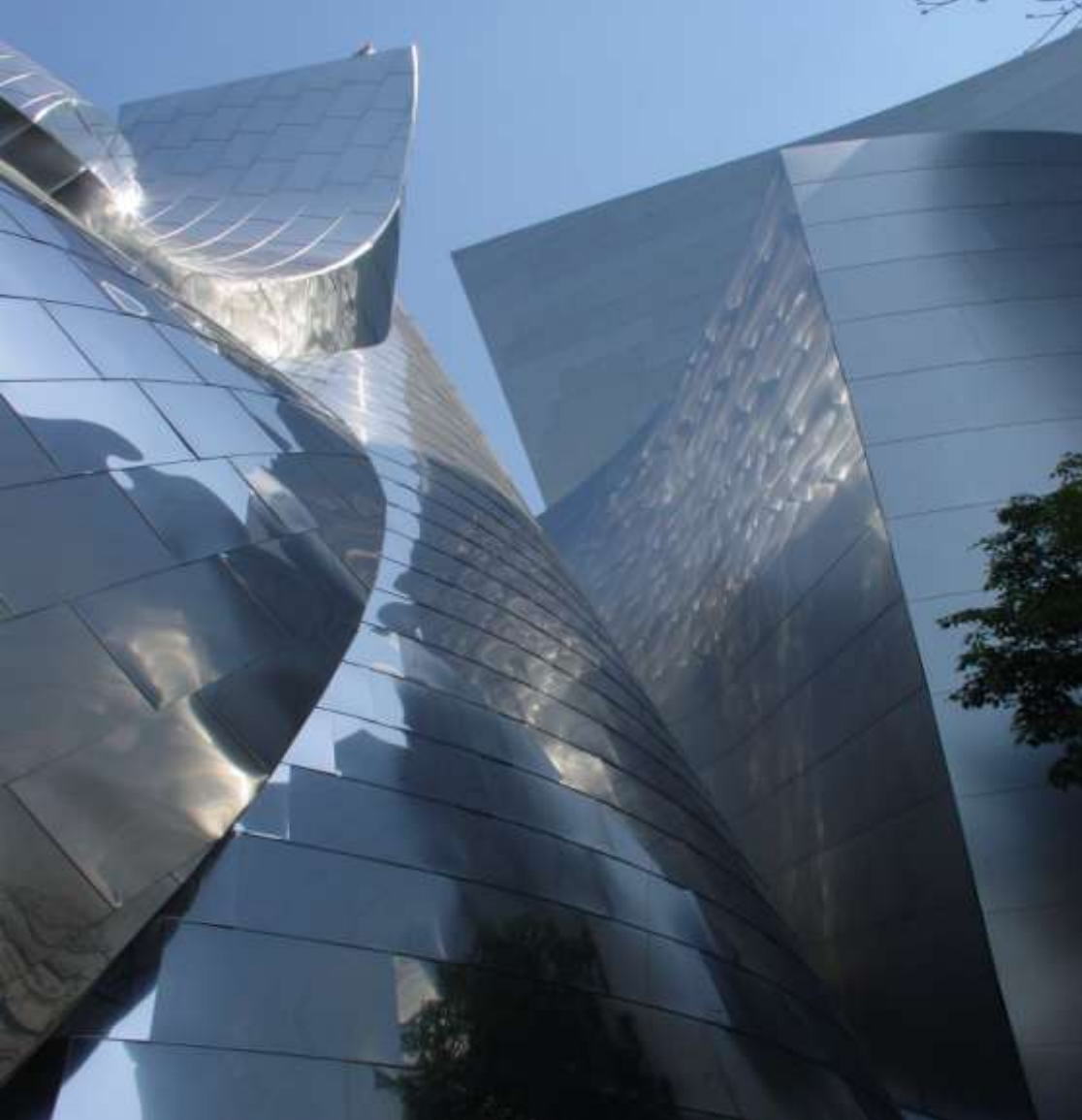
Flat lock seam stainless steel panels Disney Concert Hall, Los Angeles
