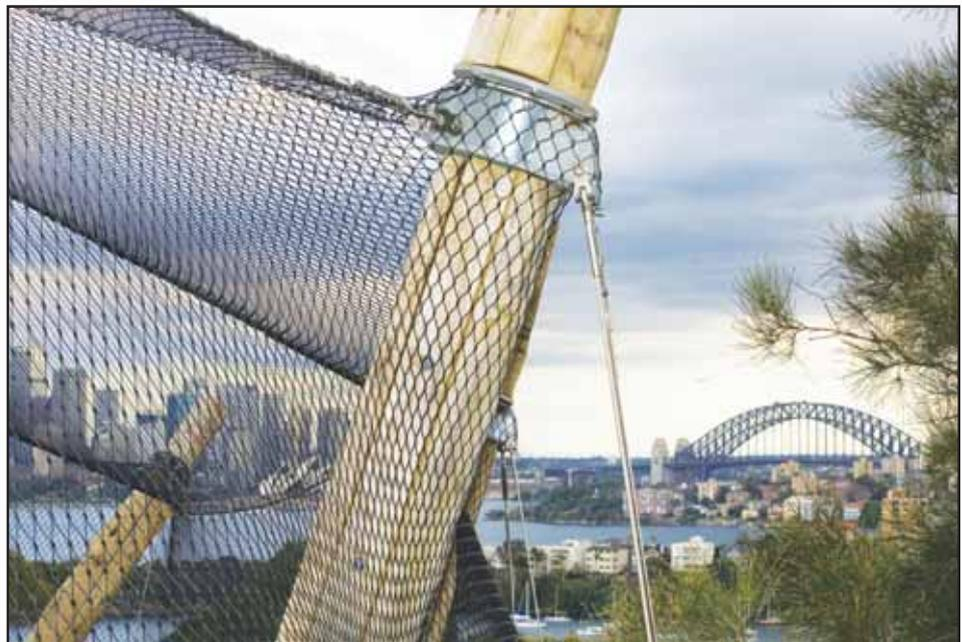
A non-climbable wall with a removable curtain, allows both spaces to function as one large paddock. This enables introduction of new chimpanzees into the compound and helps manage the apes' complex behaviour patterns.
